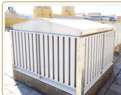
Louvers and sand trap
